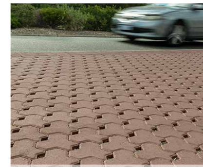
Permeable parking bays
